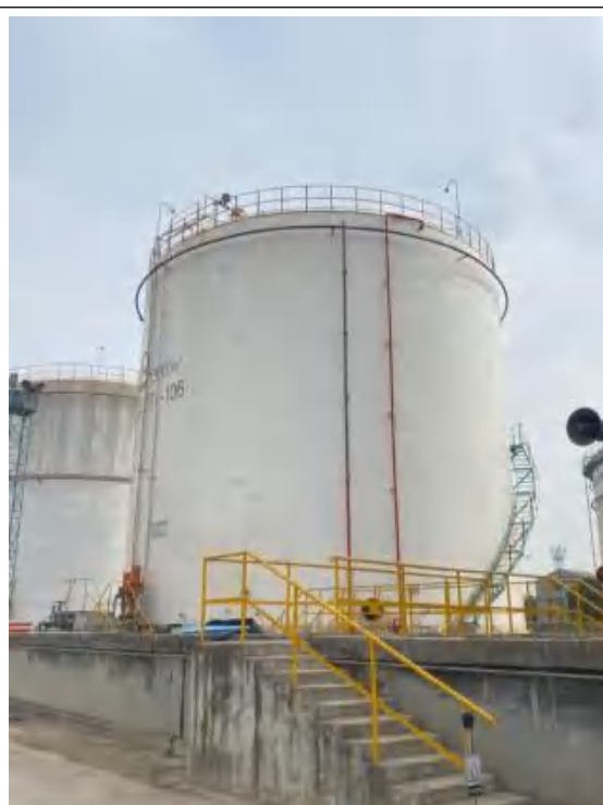
江边罐区原油罐改为石脑油罐
