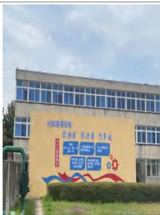
江边罐区防爆墙
